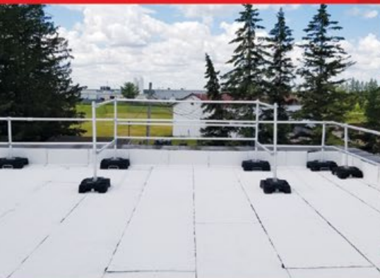
VSS Compact Guardrail and snow removal guardrail
