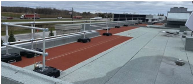
HVAC unit - VSS Compact
