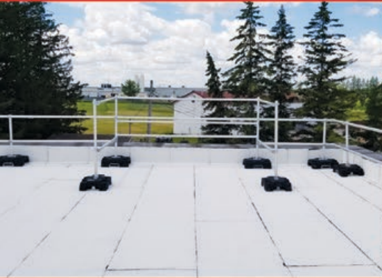
VSS Compact Guardrail and snow removal guardrail
